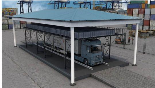
**Figure 1.8.** | large area detectors of Decision Sciences for the scanning of commercial trucks. Reproduced from [58].
