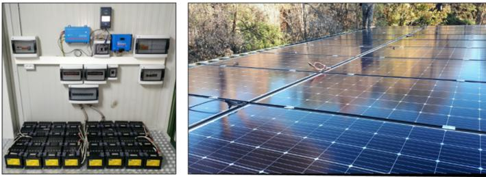
**Figure 3.11.** | Battery system installed inside the container (left) and solar panels mounted on the roof (right).
